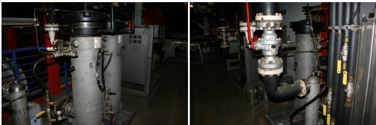
Figure 2.6/2.7: Pictures of the Helium Gas Recycler Sections at the National Hyperbaric Centre in Aberdeen's Saturation Diving Chamber. The left picture shows the filters that clean the Helium gas of contaminants such as Carbon Dioxide before enriching it with oxygen. On the right it shows the piping that connects the system to the dive chamber which is on the floor above. Both Pictures Copyright Hugh Finlayson (2008).
